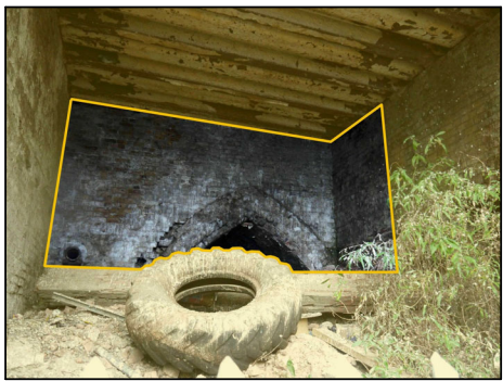
NON-LISTED STRUCTURES MASKING THE LISTED CROSS ARCHES TO BE REMOVED IS SHADED YELLOW.
