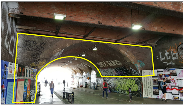
EXTENT OF NON LISTED ARCH TO BE DEMOLISHED HIGHLIGHTED IN YELLOW
